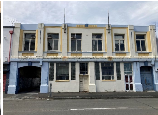
Deteriorating building. Lowe St
