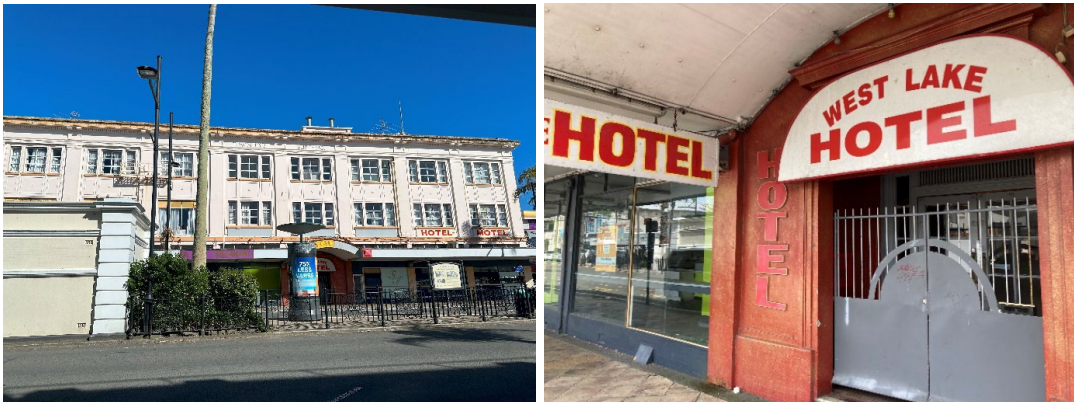
Former Westlake Hotel. Corner Gladstone Rd and Peel St
