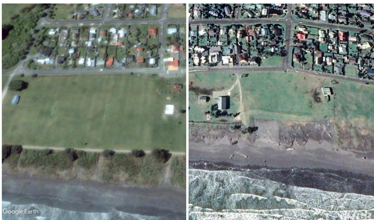
Figure 9: Coastal erosion at Carters Beach in 2003 (left) and 2019 (right) (Google Earth Pro 2003 and 2019).
