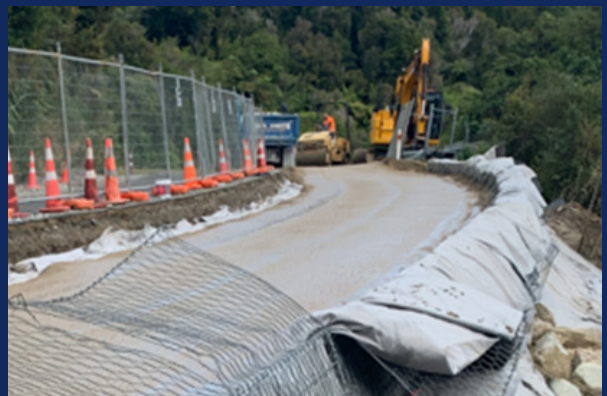
A mechanically stabilised earth (MSE) retaining wall on the Karamea Highway Photo by Buller District Council
